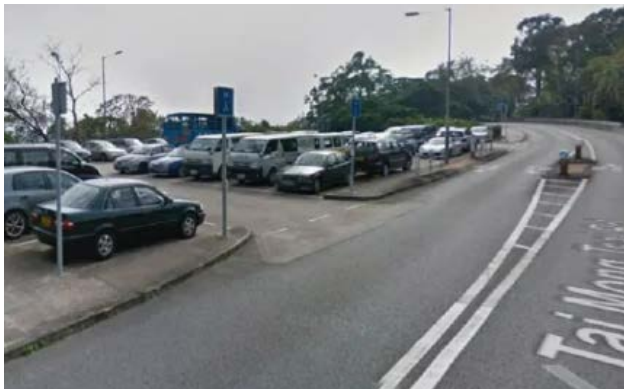
Conventional asphalt surfaces
